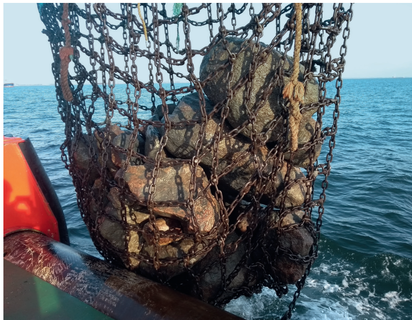
FIGURE 8 Recovery of the boulder removal net.
