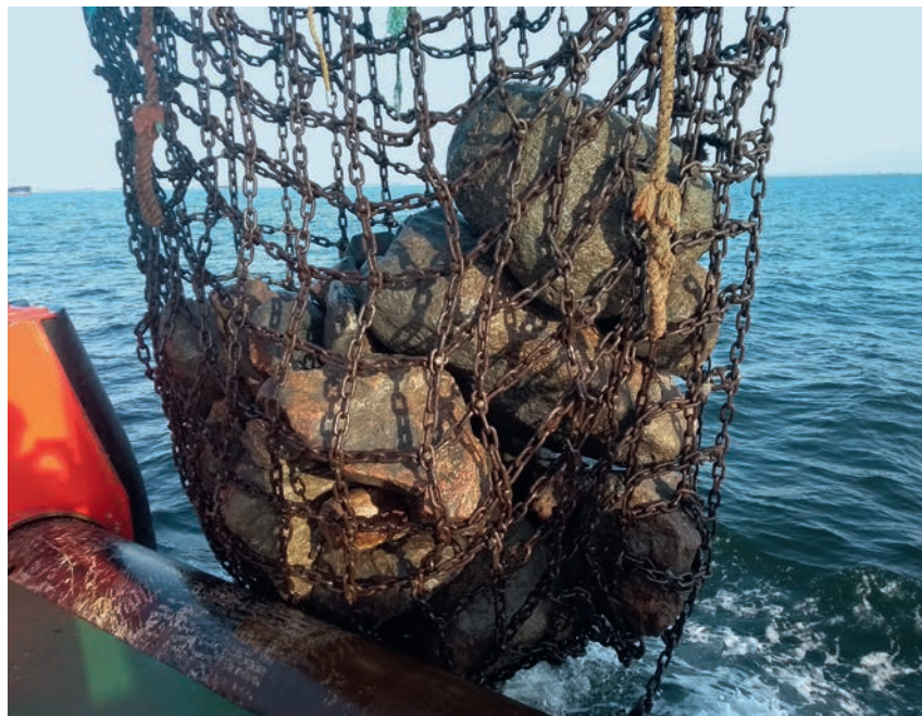
FIGURE 8 Recovery of the boulder removal net.
