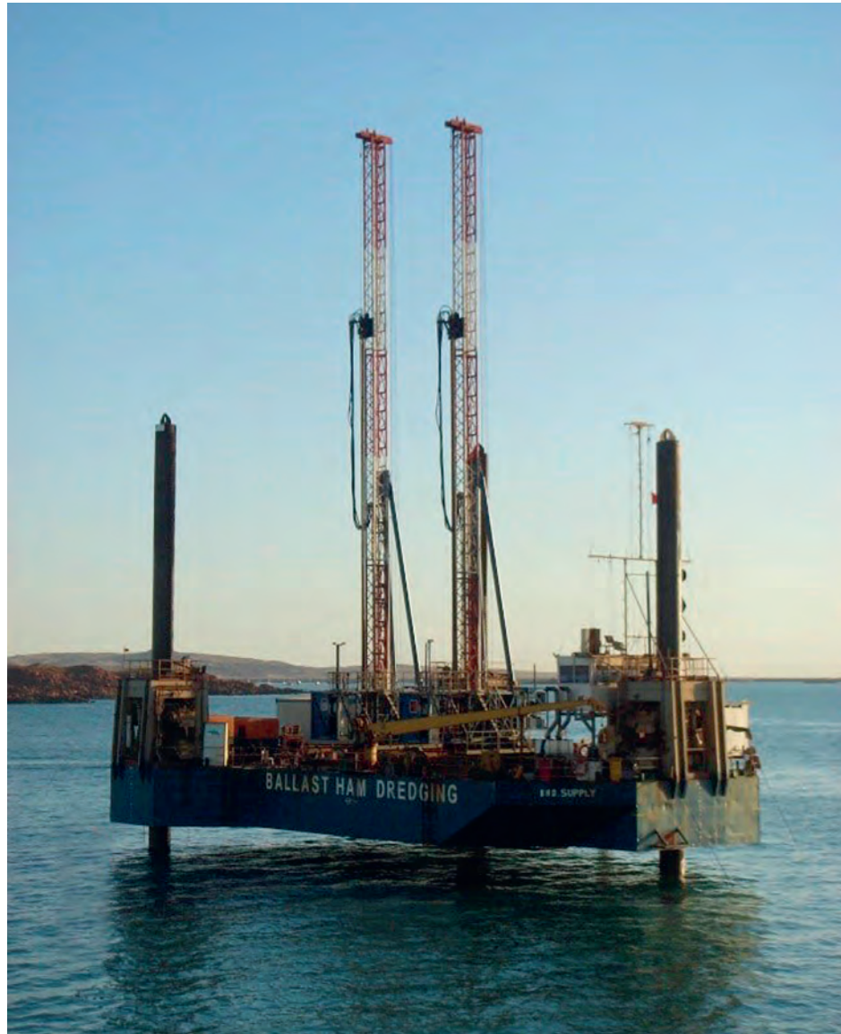
FIGURE 2 Jack-up barges are often used for site investigations.
