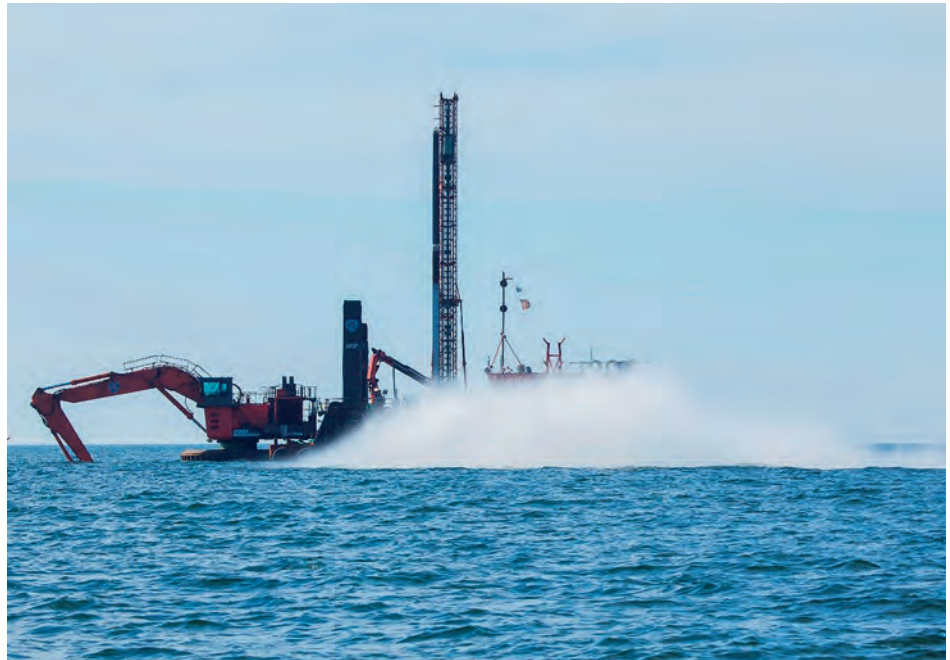
FIGURE 1 Drilling and blasting is a specialised operation. Photo @ Anko Bos.
