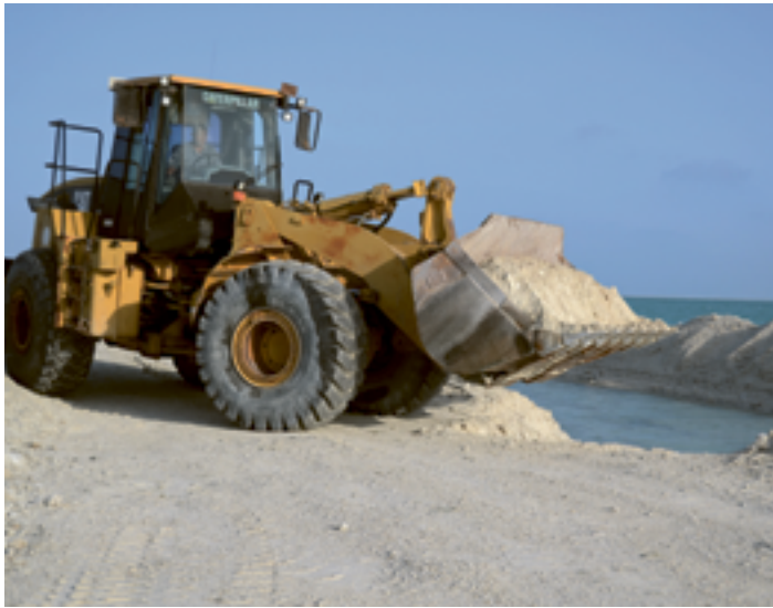
FIGURE 5 Excavation of tidal channels along causeway.
