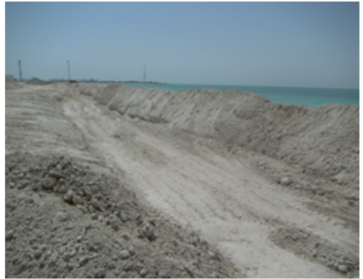
FIGURE 6 Completed tidal channel prior to planting.
