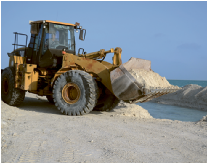
FIGURE 5 Excavation of tidal channels along causeway.
