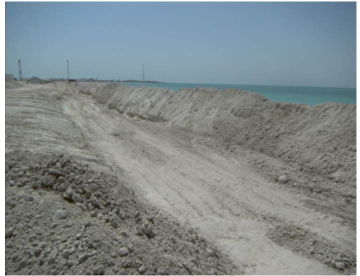
FIGURE 6 Completed tidal channel prior to planting.
