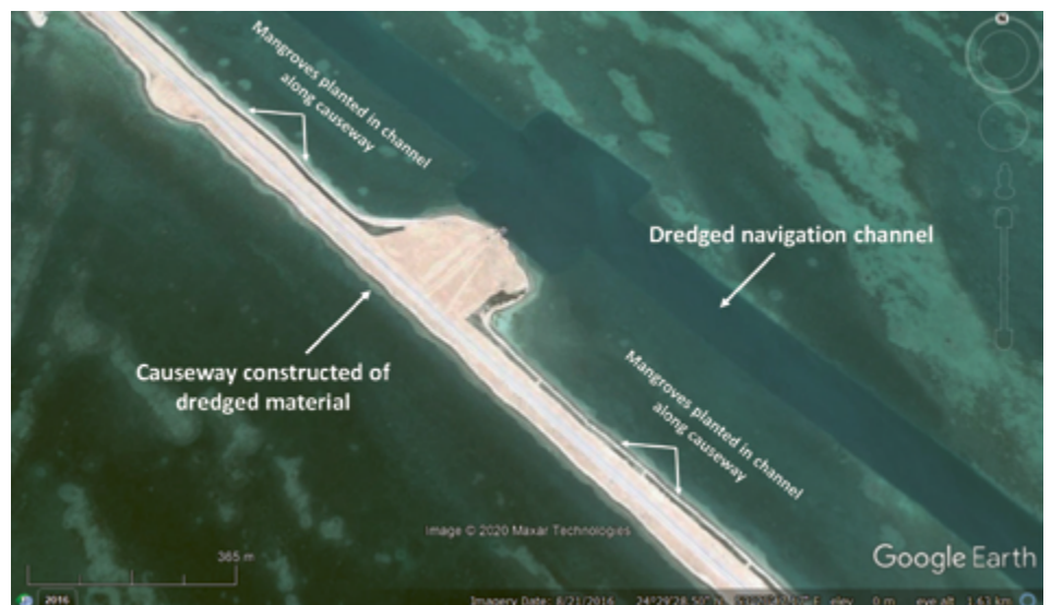
FIGURE 7 Aerial view of causeway, tidal channels and navigation channel. Map data: Google, image © 2020 Maxar Technologies.
