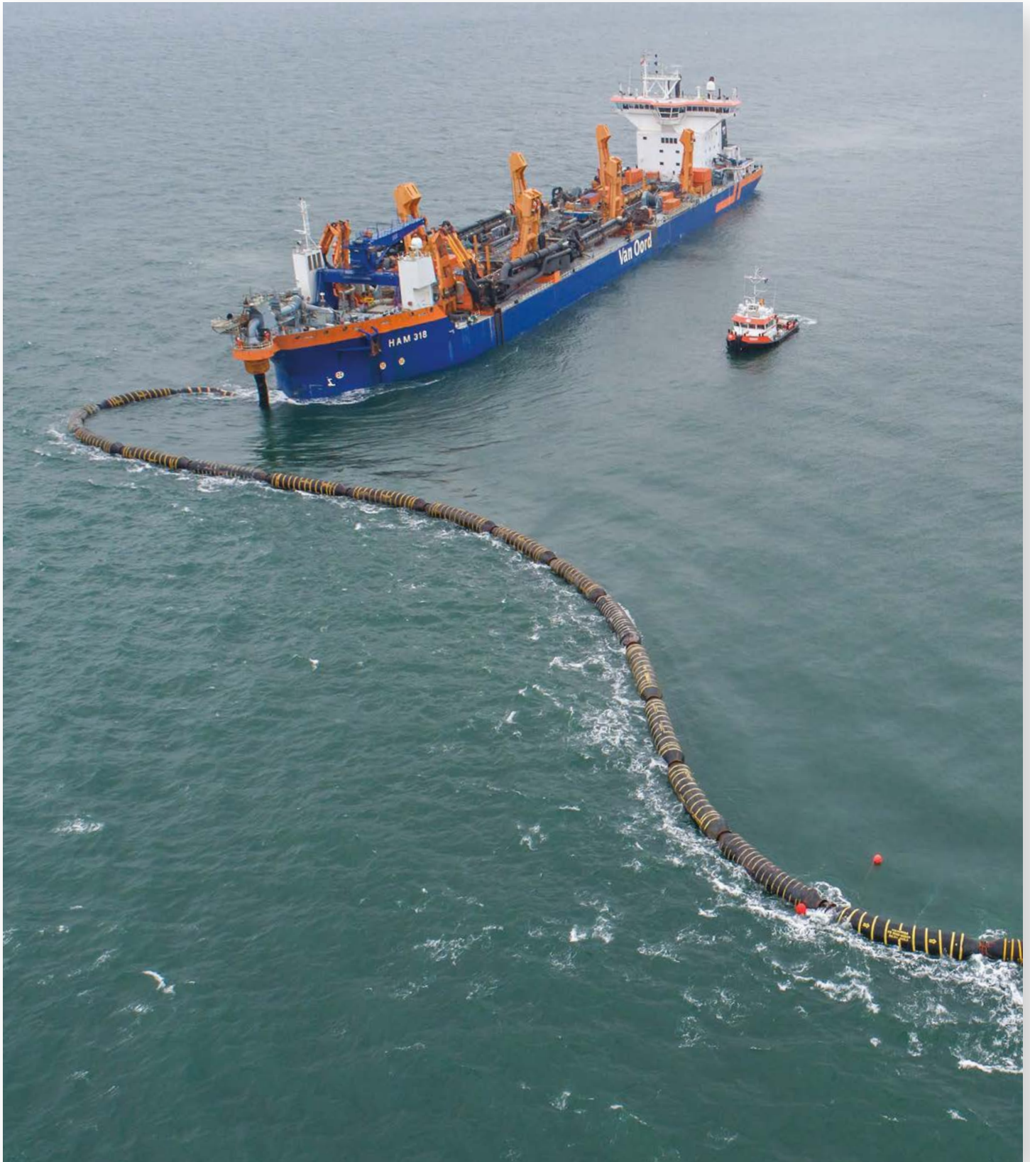
FIGURE 9 Floating pipeline delivering sand to the shore from an offshore site.
