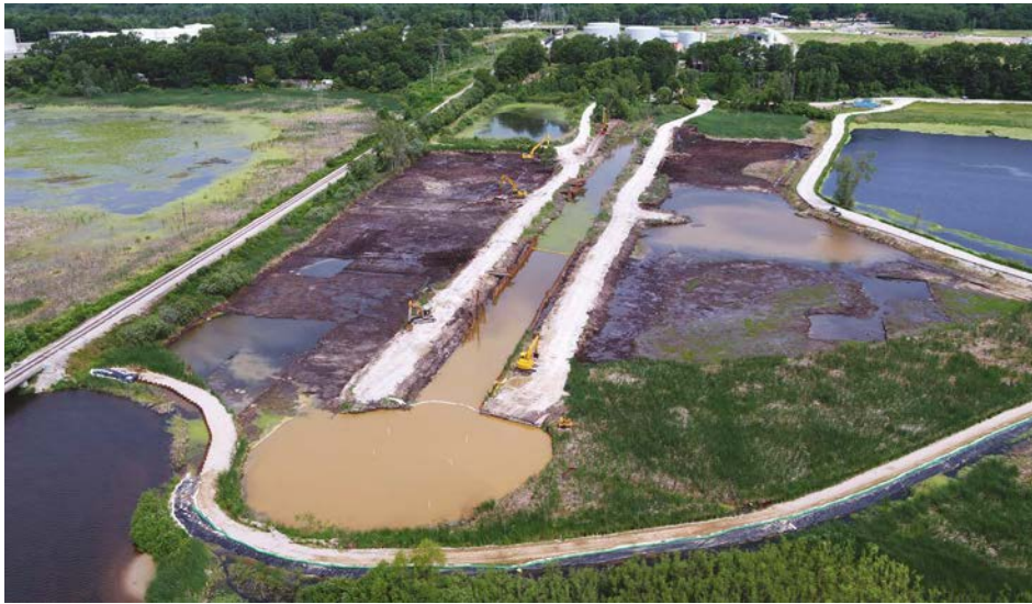
FIGURE 1 Contractors staging native plantings in emergent wetlands.
