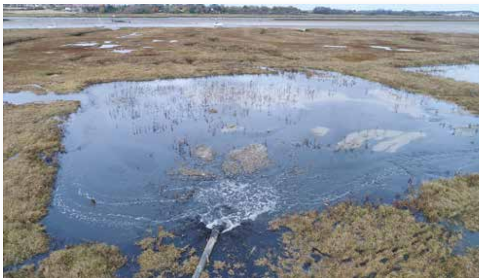
FIGURE 7 Depositing dredged sediment to enhance wetlands. Photo Exo Environmental
