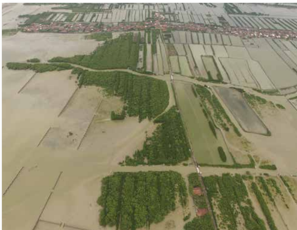
FIGURE 1 The restoration of an eroded coastline in Northern Java, Indonesia. Photo EcoShape
