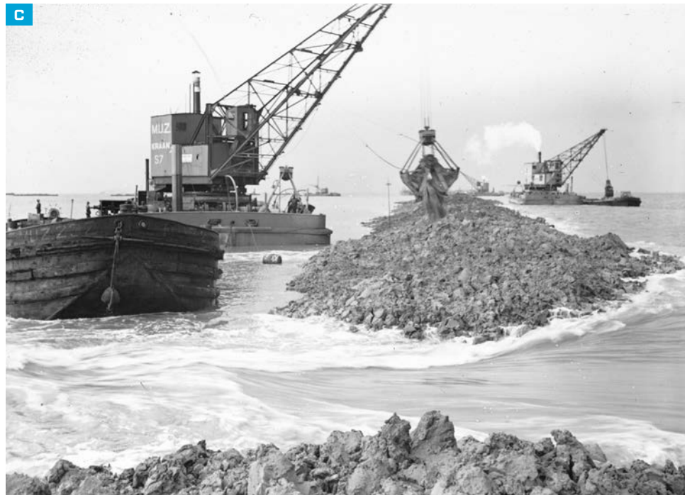
(A) The bucket dredger Arnhem from the Adrian Volker company. Bucket dredgers were introduced in the 1860s. Photo courtesy of the National Dredging Museum, Sliedrecht. (B) The development of the Port of Surabaya, Indonesia (then the Dutch Indies) in the 1920s. Photo courtesy Van Oord. (C) 27 May 1932, a day before the closure of the Afsluitdijk dam that closed off the Zuiderzee, creating the IJsselmeer.
