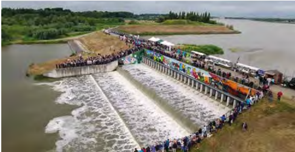
An aerial view of the Meiresluis – the sluice named after Patrick Meire in Kruiabeke, Belgium – at its inauguration on 24 June 2017.
