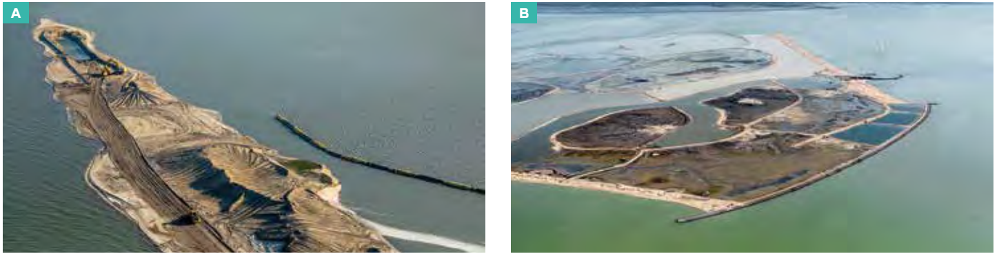
FIGURE 4 Construction of sandy beach and dunes (A) as well as the rock revetment at the west side of the island (B).
