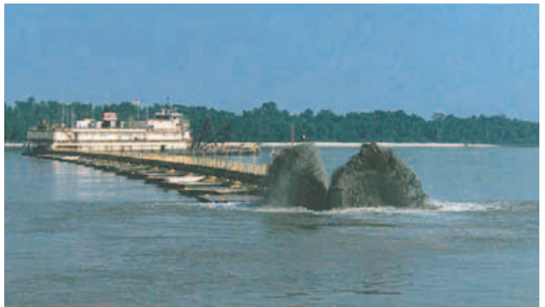
Dustpan dredger at work in a river.
