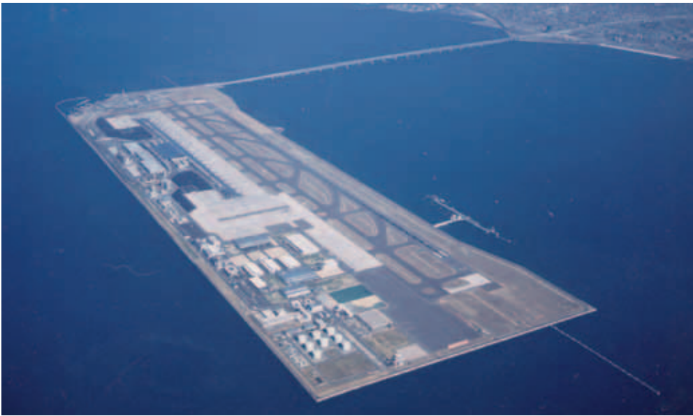
Kansai International Airport, Japan is constructed on an artificial island made by dredging.
