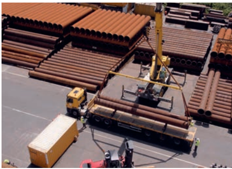
Figure 2. The team chose to proactively eliminate the potential risks to safety by replacing accepted norms within the loading process with certified alternatives.
