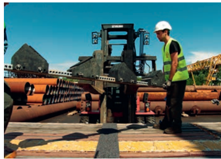
Figure 3. To begin loading pipes onto the truck’s flatbed, bottom section cradles are placed atop an anti-skid mat.
