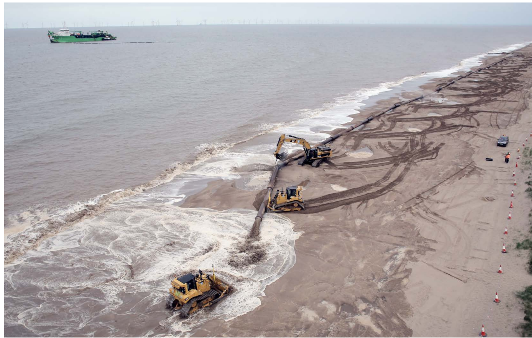
Figure 9. Lincshire Beach Renourishment project, eastern coast of the UK.
