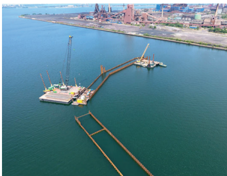
Figure 5. Construction of the 6.2 hectare Engineered Containment Facility. Photo McNally Construction Inc.
