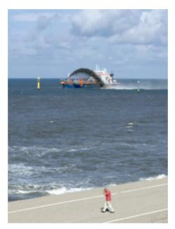
Figure 2. Twenty million cubic metres of sand were placed on the Dutch coastline to strengthen the Hondsbossche and Pettemer Sea Defences in northwestern Holland. The sailing distance to and from the extraction site must also be considered in evaluating the C0, footprint.
