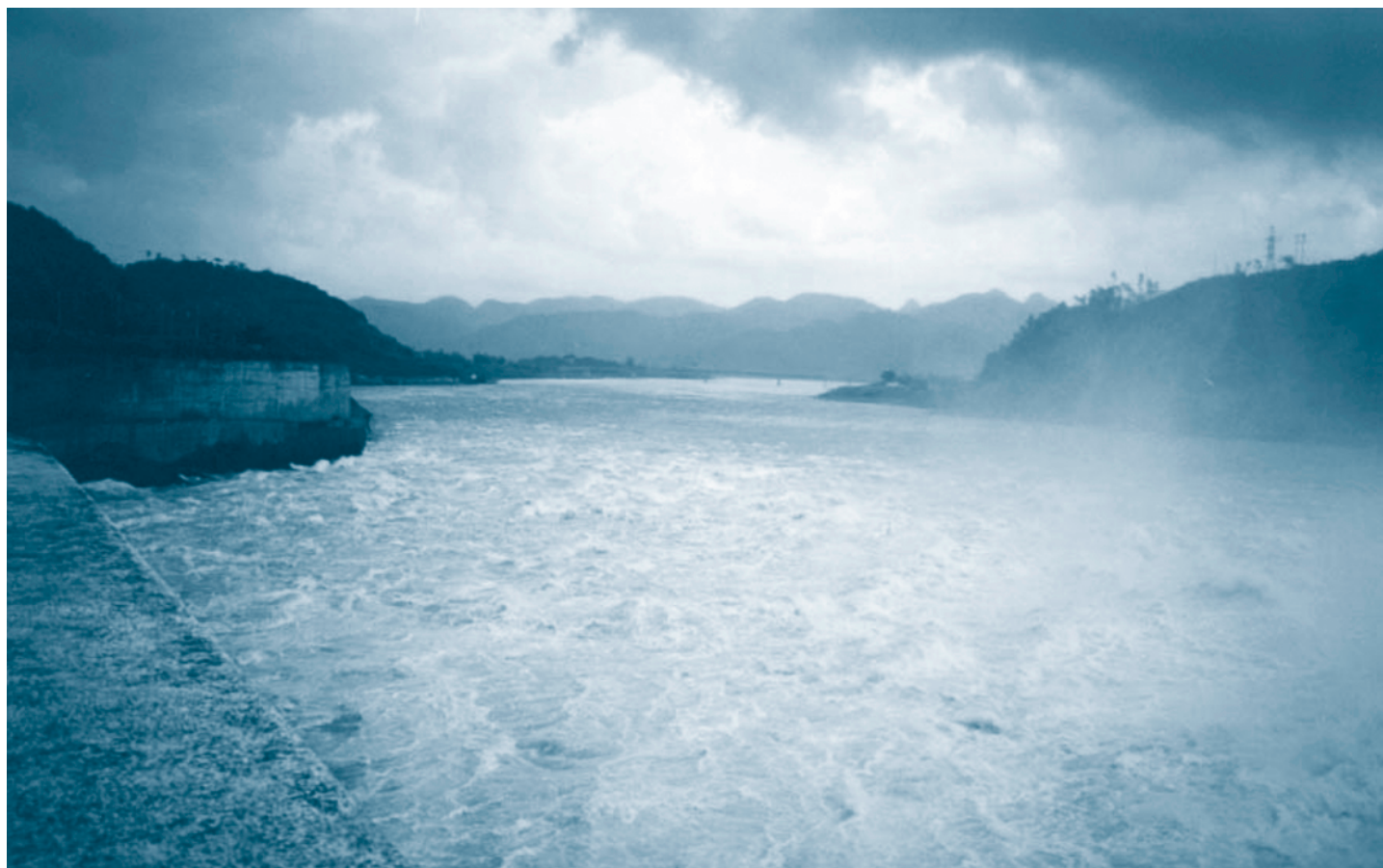
Figure 6. Da River downstream from the Hoa Binh Dam at 500 m 3 /s, with one gate of eight opened.
