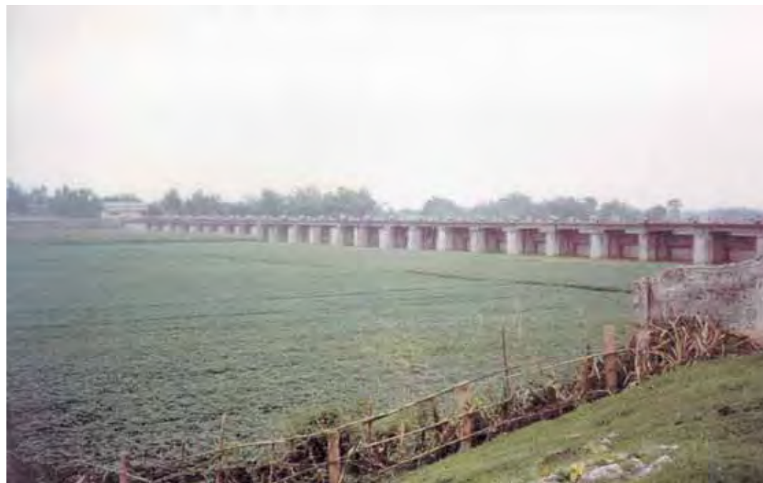
Figure 5. Van Coc's Flood Diversion Structure with 25 gates; and a spillway of 8.6 km length carrying together a maximum diversion of 5,000 m 3 /s from the Red River into the Day River.
