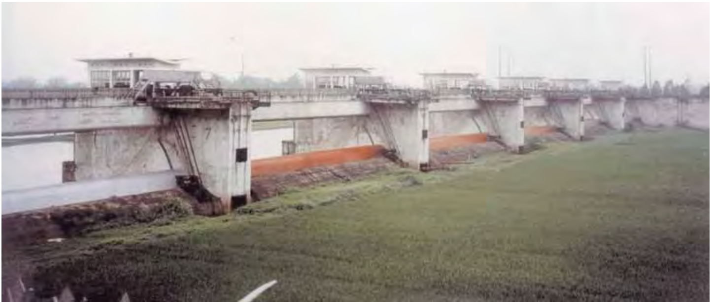
Figure 4. The Day Barrier built in 1937, with six moveable weirs with a maximum capacity of 5,000 m 3 /s.
