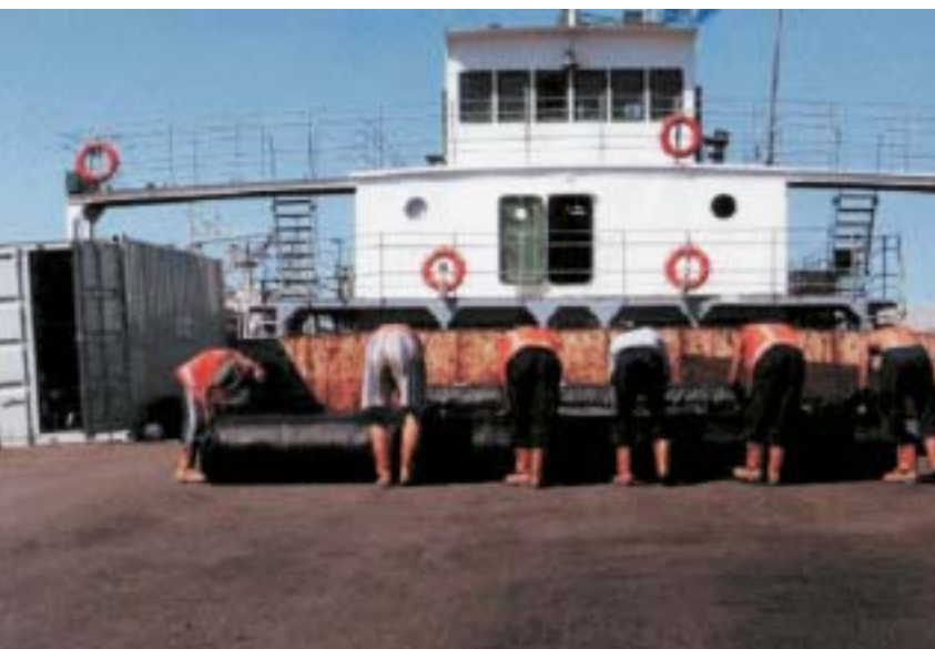
Figure 6. Unrolling the geotextile mats.
