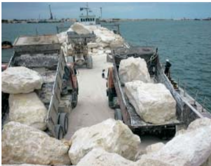
Figure 8. The transfer of rock to the Bautino stockpile was done with local trucks.
