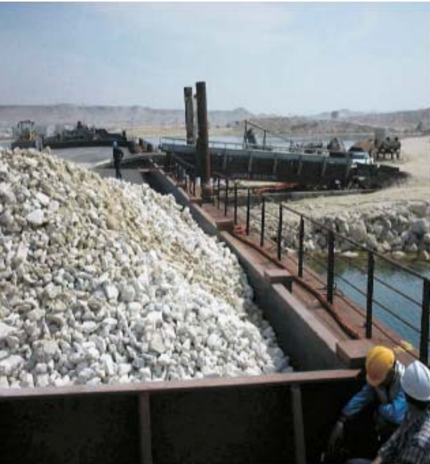
Figure 9. A total quantity of more than 200,000 tonnes of rock was produced from the quarries and stockpiled in Bautino.
