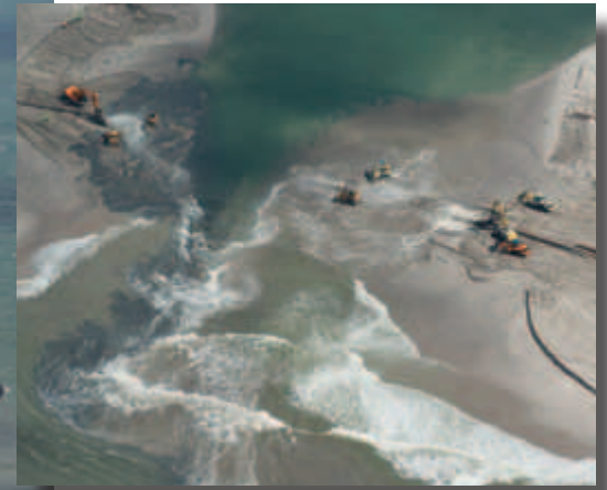
Figure 28. Closure of the soft sea defence on July 11, 2012. TSHDs from far left to right: Vox Maxima , Prins der Nederlanden , Crestway and Ham 317 . Insert: Closing the gap, the land-based equipment spreading sand.
