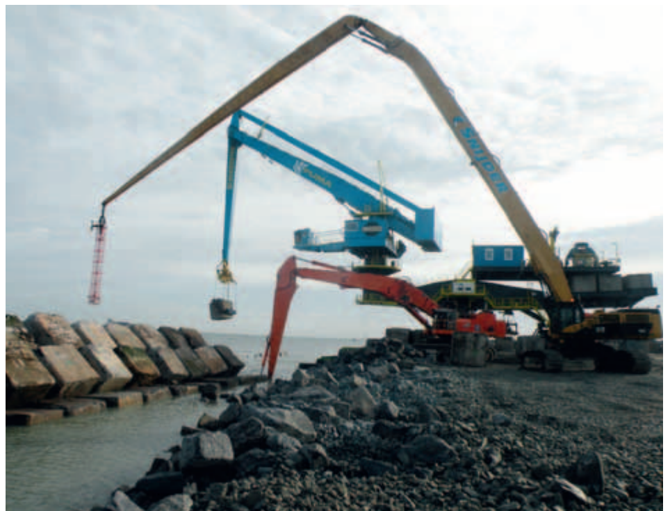
Figure 9. Three specialised land-based machines used at Maasvlakte 2: Blockbuster, Hitachi 1200 and Condor.
