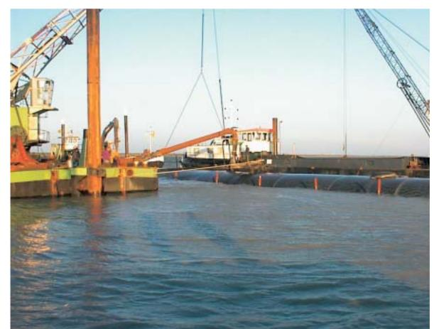
Figure 2. The geotubes made of geotextiles are filled with a water-sand mixture.
