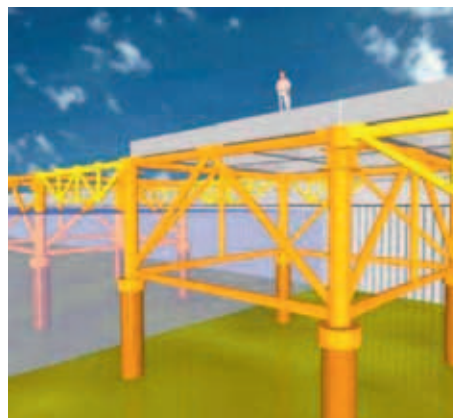
Figure 5. Containerland: slabs in terminal load (left), Maxisteck (right): Jetty for liquid bulk, transshipment, piles as foundation piles or dolphins.
