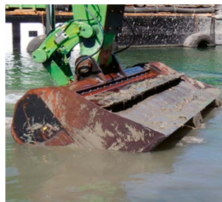
Figure 4. A visor bucket in being utilised for dredging at Valdemarsviken fjord.
