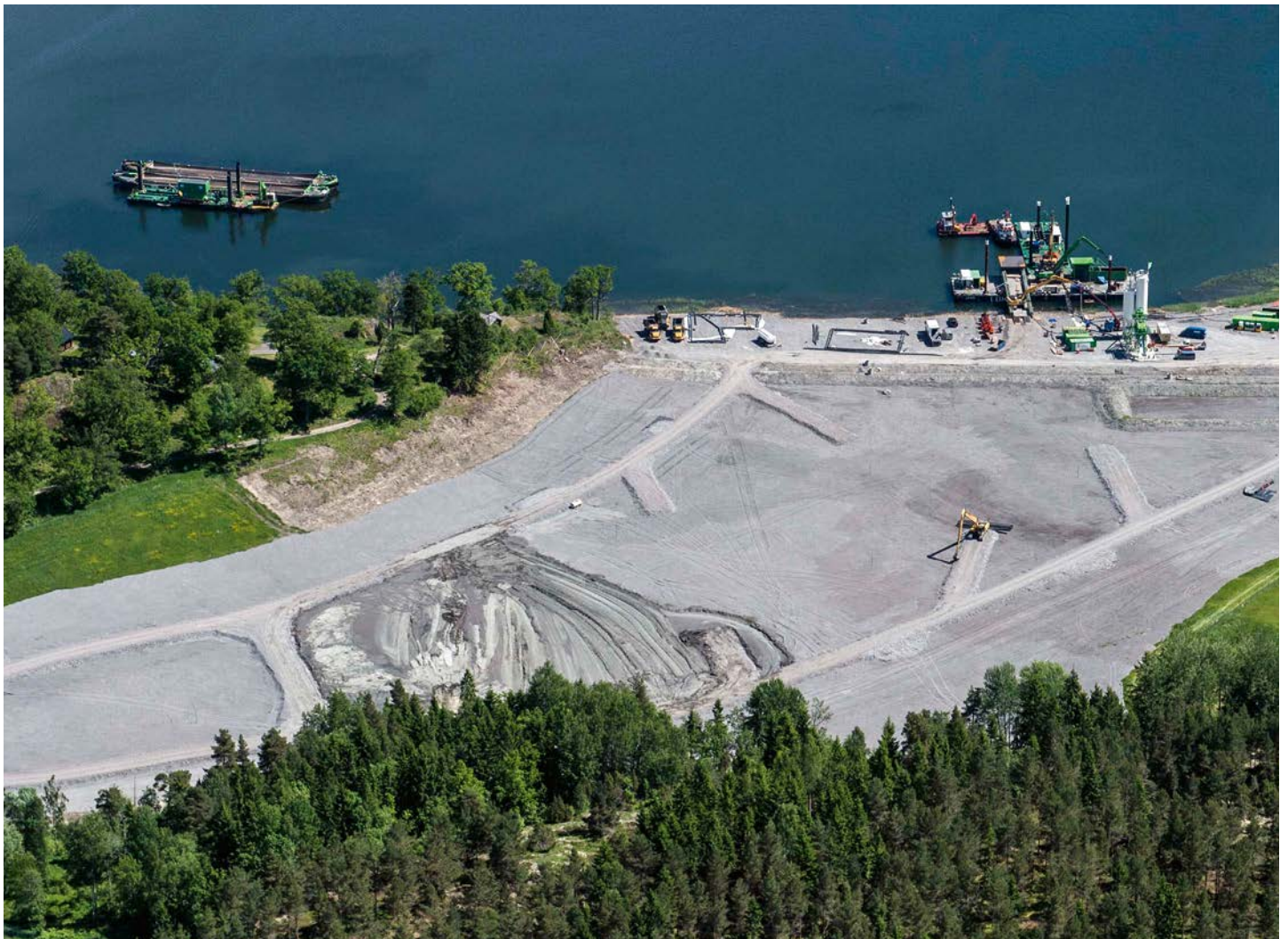
Figure 9. An aerial view of the Grännäs backfill area near completion.
