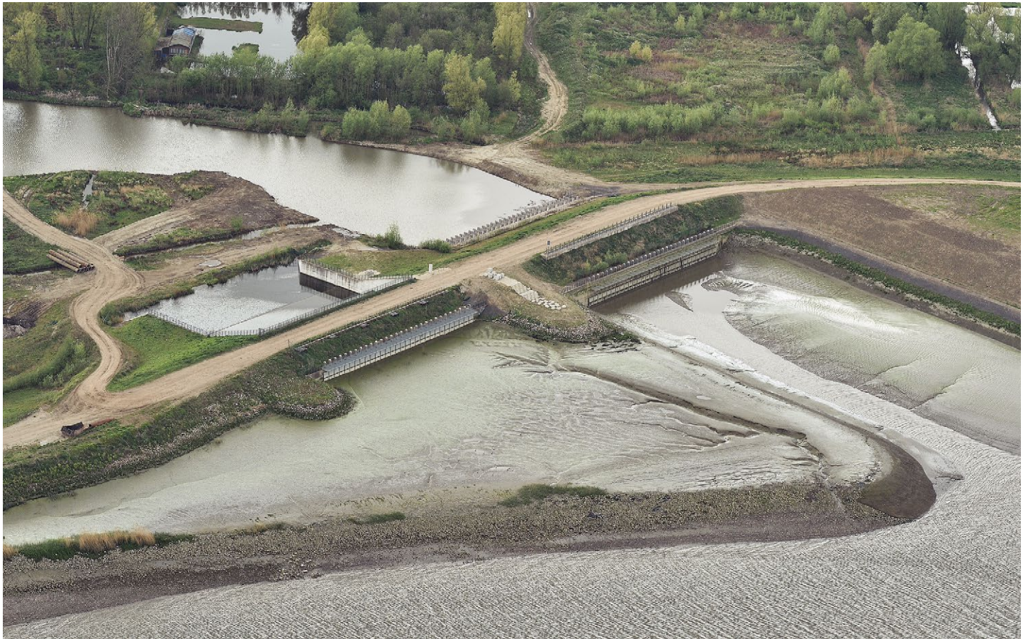
Figure 7. Close up view of the sluice system in the northern part of the project connects the project site with the River Scheldt. The sluice will reduce the tidal range that comes into the area, thus creating a Controlled Reduced Tide. Making the sluices, lowering the dike next to the river and building the new ring dike land inwards are the main dredging operations in this project.
