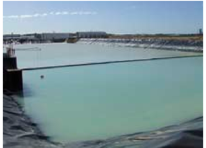
Figure 8. The settlement pond showing water quality monitoring and equipment (left) and silt screen in the middle.
