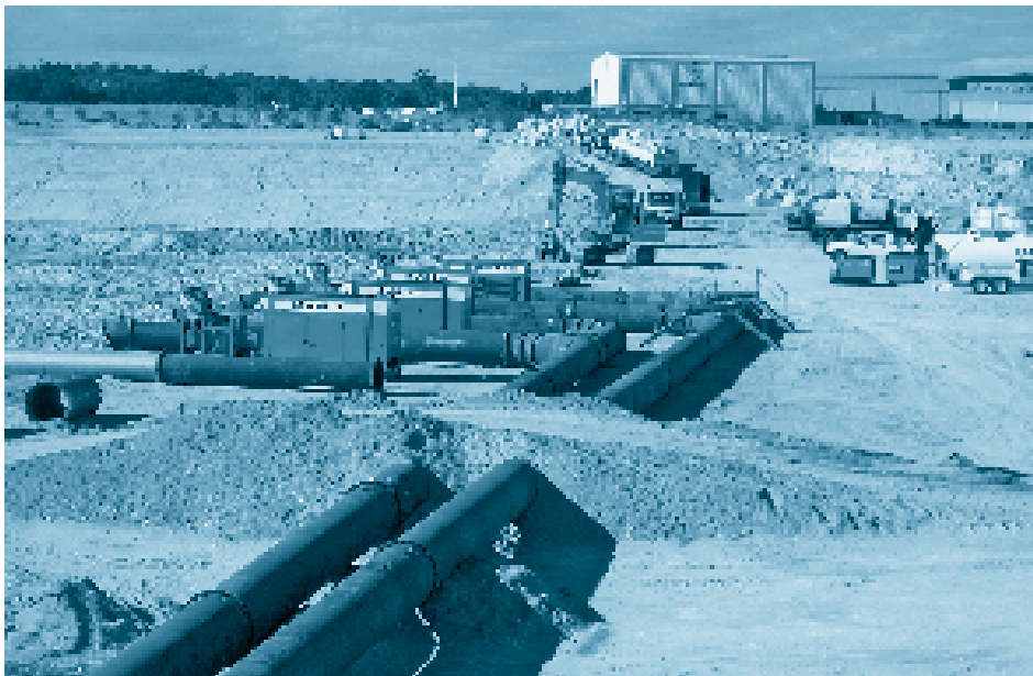
Figure 5. Another view of the Van Heck pumps from the reclamation area.
