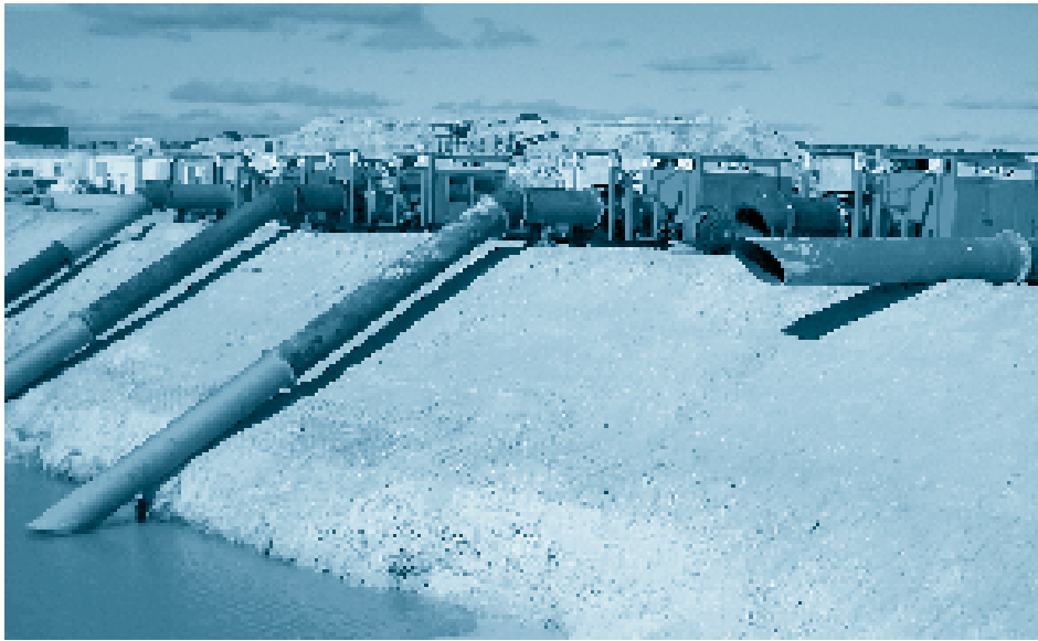
Figure 4. Four Van Heck pumps were used to pump the tail water from the reclamation area into the settlement pond.
