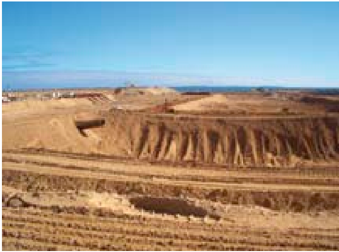
Figure 6. Preparations of the reclamation area and the initial settlement pond.
