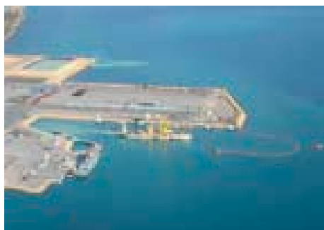
Figure 1. An aerial overview of the Australian Marine Complex site in Jervoise Bay, Western Australia.
