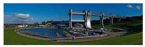
Figure 19. The Falkirk Wheel a rotating boat lift in Scotland, connects the Forth and Clyde Canal with the Union Canal. The lift, named after the nearby town of Falkirk, opened in 2002.
